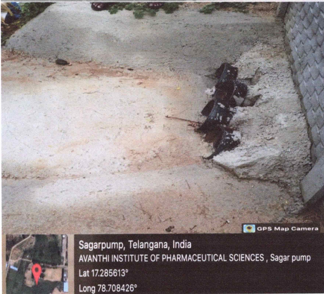
Proper drainage system
